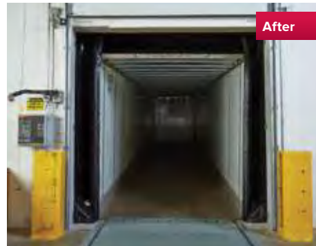
Eclipse header seals the gaps, blocks the light
